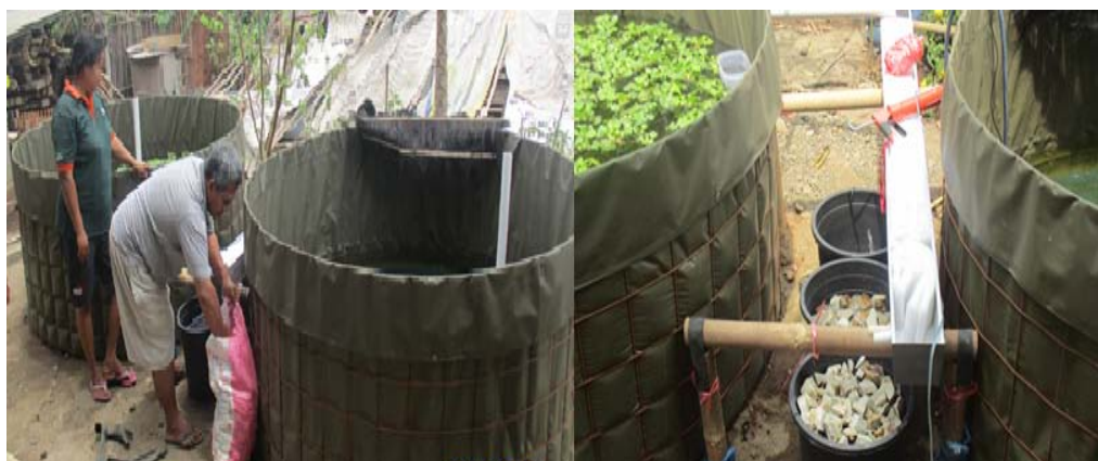
Gambar 5. 11 Set Up penjernih air kolam terpal
